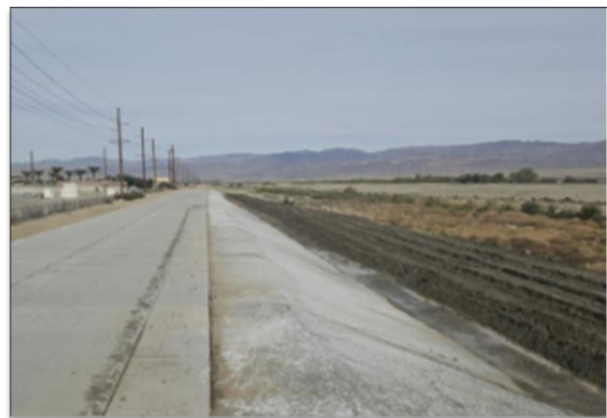
Ave 54 to Airport wetside backfill.
