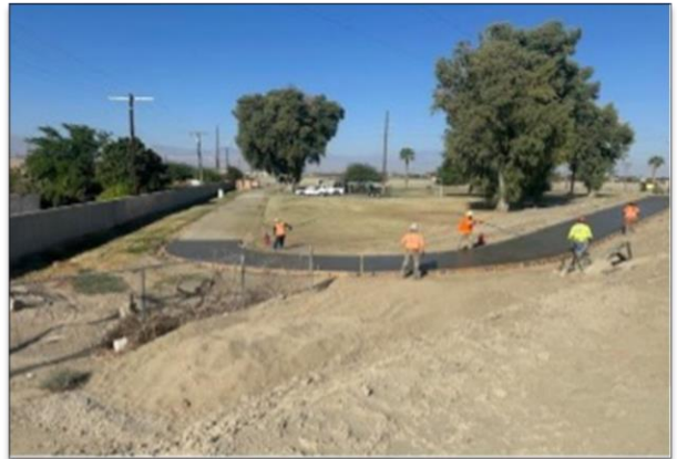
Placing Jointed Plain Concrete Paving at Sierra Vista Park Connector.
