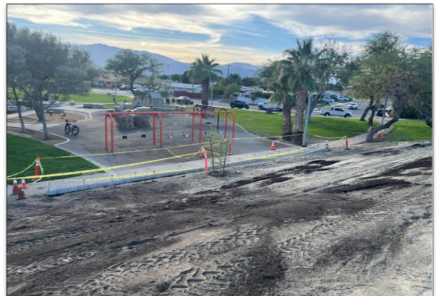
Irrigation and wall installation at Jackson Park.
