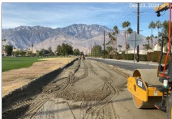
Grading and compaction along 34th Ave off-street path in Palm Springs.
