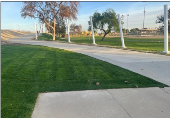
Light columns and landscaping install at Jackson Park in Indio.
