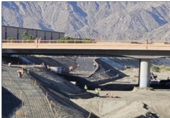
Rebar install at Jefferson Undercrossing to prep for concrete placement.
