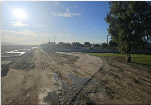
Infill formwork at Sierra Vista Park Connector in Coachella.
