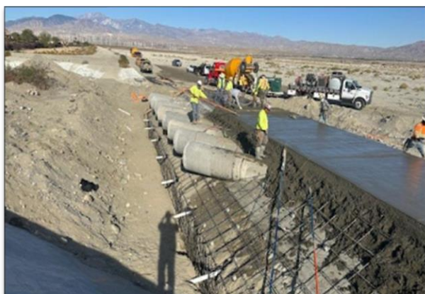
Placing shotcrete over in-channel culvert; Sunrise Way to Gene Autry
