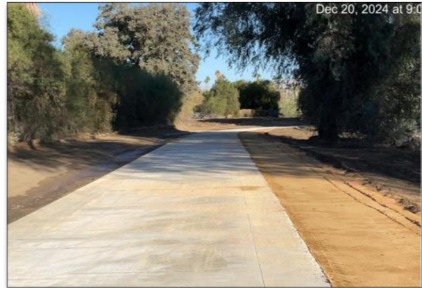
Grading 6' DG path on the dry side between west side of E Cielo and Mesquite in Palm Springs.
