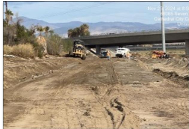
Grading and balancing dirt south of Dinah Shore.
