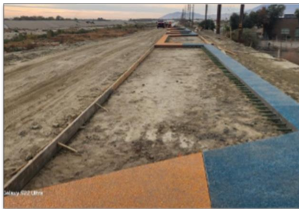
Infill formwork at Ave 54.
