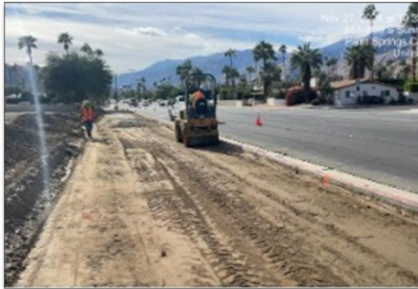
Grading and balancing dirt on the east side of Sunrise Way in Palm Springs
