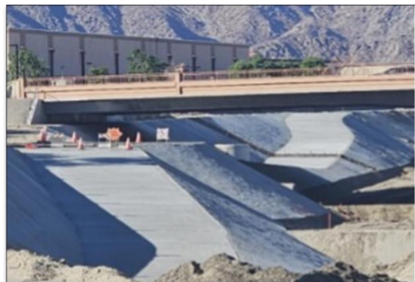
CSP curing at Jefferson Undercrossing in La Quinta / Indio.
