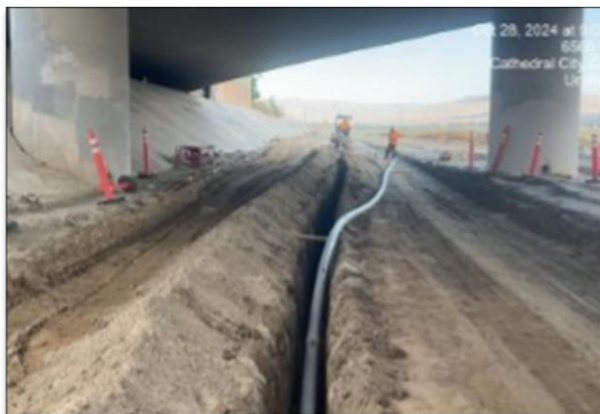
Belco onsite excavating and installing conduit south of Dinah Shore bridge.
