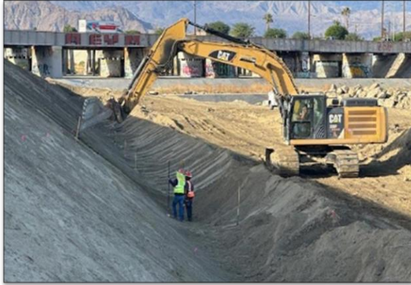
Fine grading for new concrete slope protection; Fred Waring to CONN_BUS.
