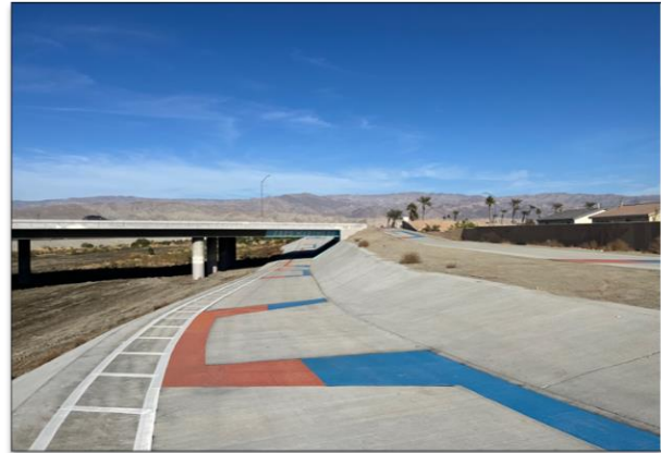
Thermo banding install at Fred Waring Drive Undercrossing.
