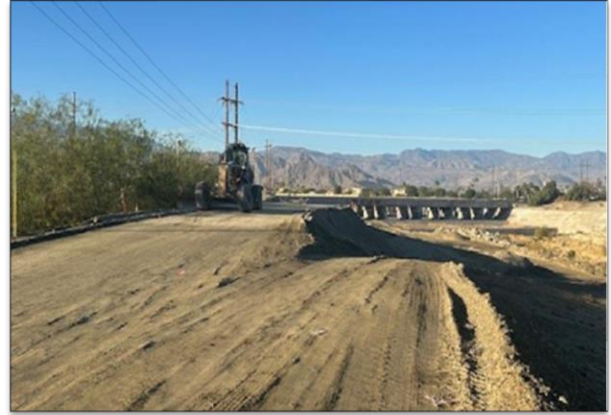
Grading subgrade for Jointed Plain Concrete Paving; Indio Blvd to CONN-BUS.
