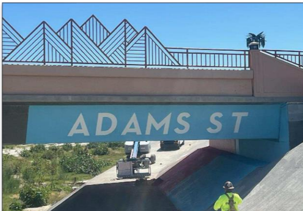
Adams Street undercrossing painted in CV Link's signature orange and blue colors.
