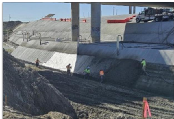
CSP placement at cutoff wall for Ave 52.
