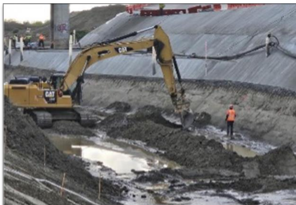
Dewatering and cutoff wall excavation continued at Ave 52.
