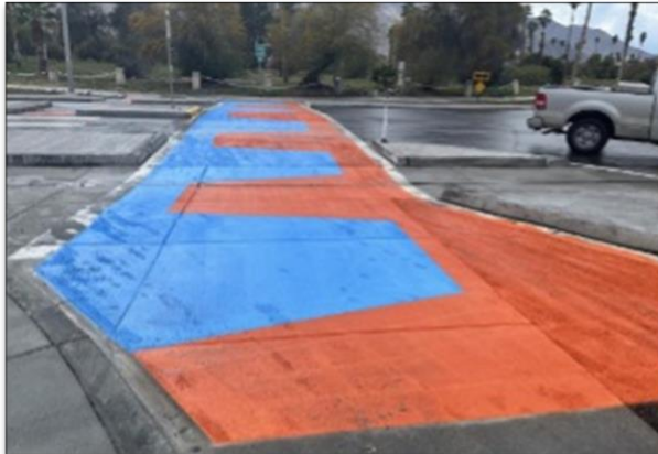
Striping upgrades to the crosswalk at El Cielo and Mesquite.
