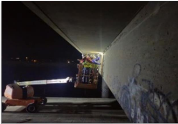
Crews remove Cliff Swallow nests at the Ave 52 bridge.
